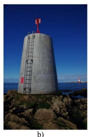
Figure 5: Application of UHPFRC, Cabon turret, Brittany, France, 4.2 m<sup>3</sup> UHPFRC applied by helicopter, 2013, a) installation of the formwork, b) finished UHPFRC surface.
