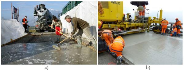
Figure 3: Application of UHPFRC. a) Bridge over river la Morge, Switzerland 6 m<sup>3</sup>, 2004, photo Alain Herzog, b) Chillon Viaduct, Switzerland– 2 x 1200 m<sup>3</sup> – 2014/2015.
